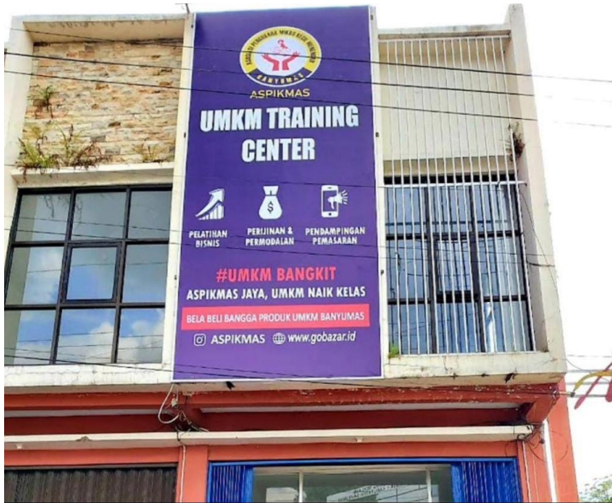
Gambar 1. Gedung UMKM Training Center ASPIKMAS
